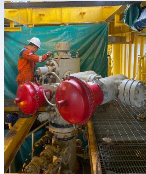
Wellhead Installation and Maintenance Services
